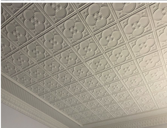
Figure 14. Example of decorative pressed metal ceilings (Image: Urbis June 2023)
