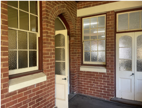
Figure 10. Exterior door and window detail to ground floor. (Image: Urbis June 2023)
