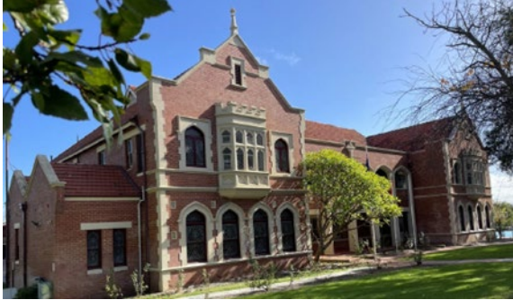
Figure 5. Exterior Loreto Convent Building showing northern wing (1931) and southern wing (1940). Webster Street elevation. (Image: Urbis June 2023)
