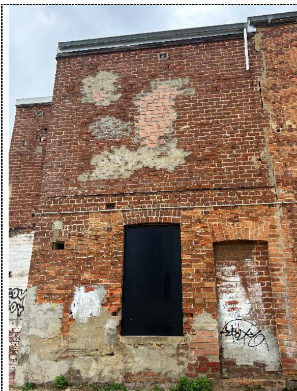
Figure 17. Upper storey addition to the south western end of Pearl Villa – contrasting brickwork.
