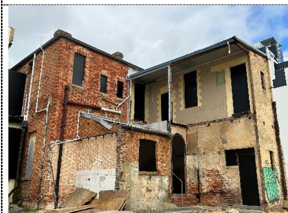
Figure 18. North and western elevations of Pearl Villa clearly showing vulnerable condition of the north elevation of Pearl Villa following the removal of non-original elements.
