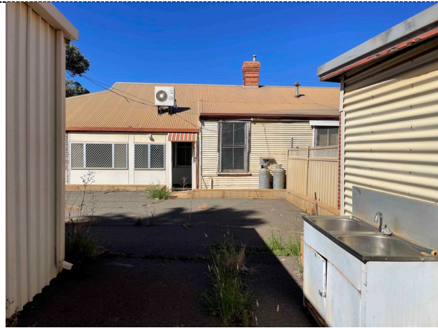
Figure 9. View of rear lot of Police Station & Quarters (fmr) looking south
