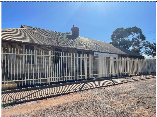
Figure 7. Exterior view of Police Station & Quarters (fmr) from Piesse Street
