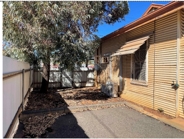
Figure 18. Police Station and Quarters (fmr) - View of east elevation
