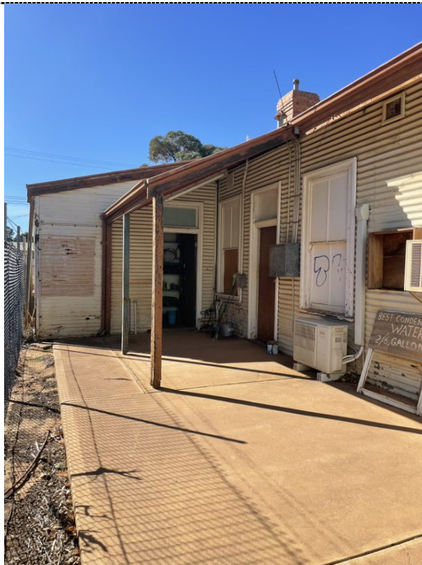
Figure 15. North elevation verandah of the Police Station.
