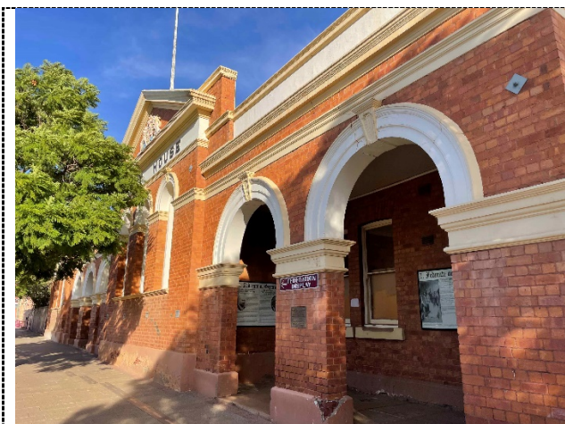
Figure 20. Court House (fmr) - North elevation of Court House showing central 'Court House' gable flanked on either side by colonnades with classical details. The west portion was constructed for the GWS office.
