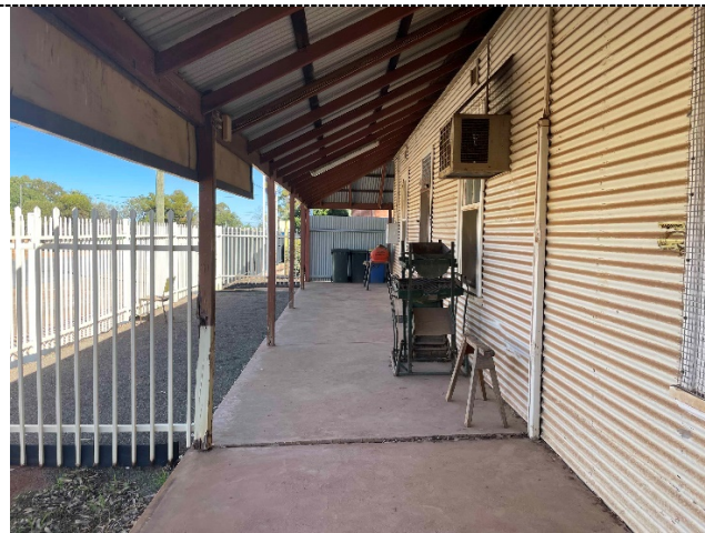
Figure 17. Police Station and Quarters (fmr) - View looking west along south verandah
