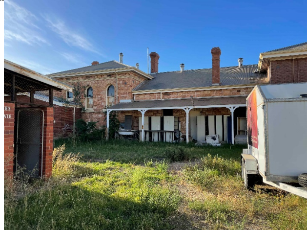
Figure 11. Rear view of Boulder Court House with nearby ancillary buildings
