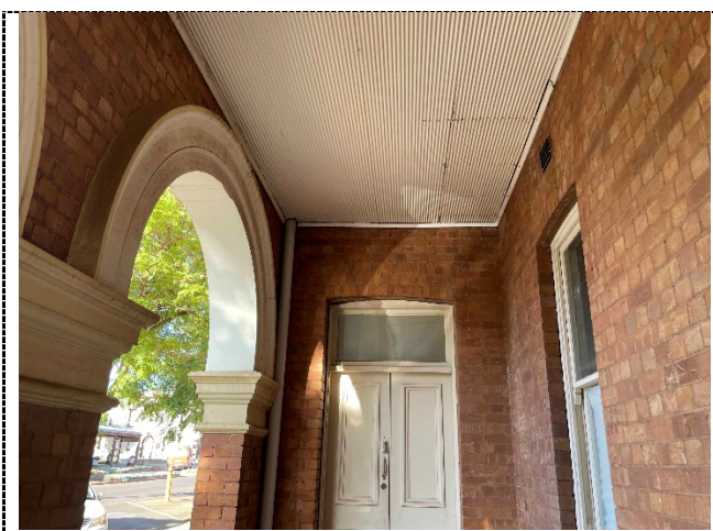
Figure 24. Court House (fmr) - Interior view of east colonnade showing typical finishes
