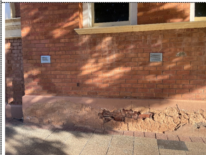
Figure 52. Court House (fmr) – Front Façade
