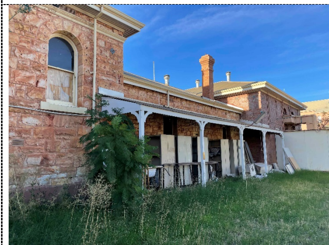
Figure 25. Court House (fmr) - Exterior view of rear (south) elevation
