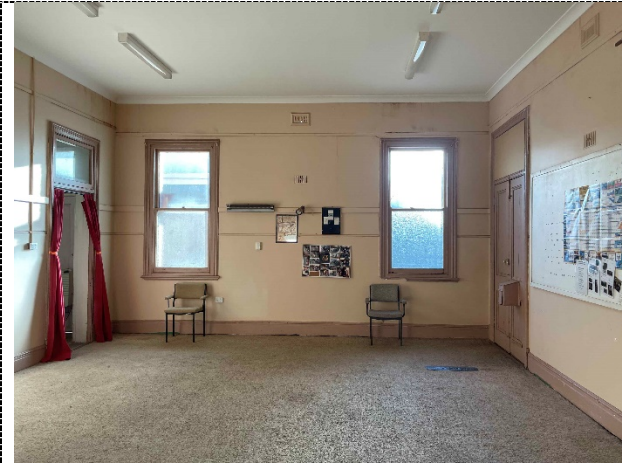
Figure 39. Former GWS Office - west wall towards entry door
