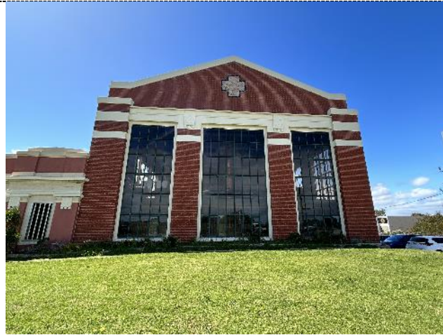
Figure 10. The large volume factory section has a classical presentation at the front elevation, with a classical balance of horizontal banding and vertical brick pilasters formed by the recessed vertical glazed panels under a gabled roof line.
