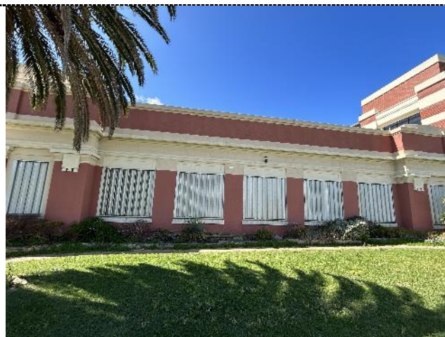
Figure 12. Providing a counterbalance to the dominant factory frontage, the single storey office building has a horizontal emphasis with a symmetrical presentation. The central entrance section is flanked by recessed wings which present with a rhythm of fenestration.
