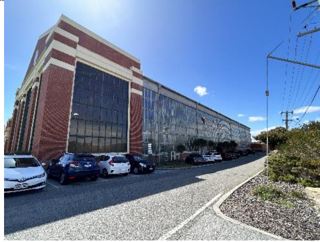
Figure 13. The south elevation of the large volume factory section is predominantly a glass curtain wall. The expansive elevation is effectively divided into bays by the prominent original rainwater heads. The fascia is corrugated metal sheeting.
