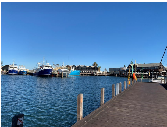
Figure 7: Boardwalk looking towards the harbour. Photograph: DPLH staff (April 2024)
