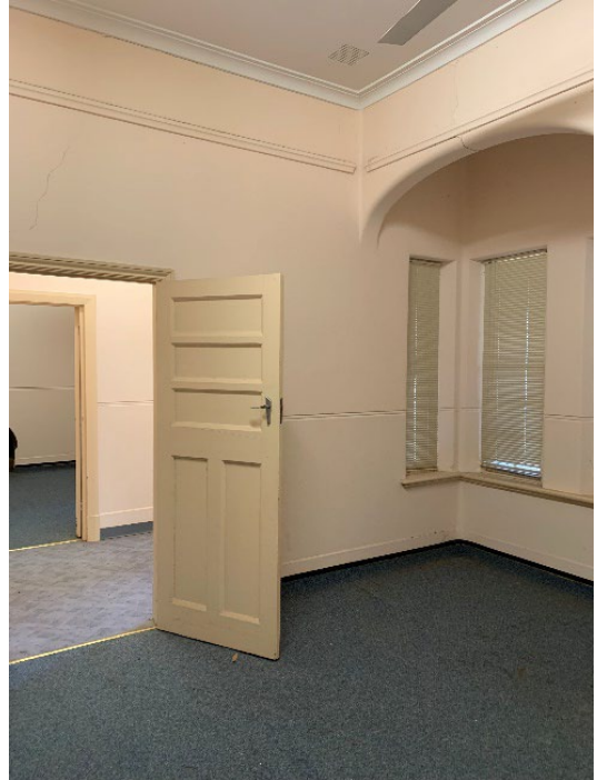
Figure 5: Southern room. Note picture rails and run moulding on walls. The hallway leads to a contemporary toilet (2024).
