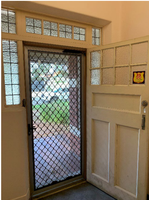
Figure 12: Internal view of front door with surrounding hammered glass windows. The jarrah door frame is likely original, though the door is c.1950s. The floor in this entrance is covered with vinyl (2024).
