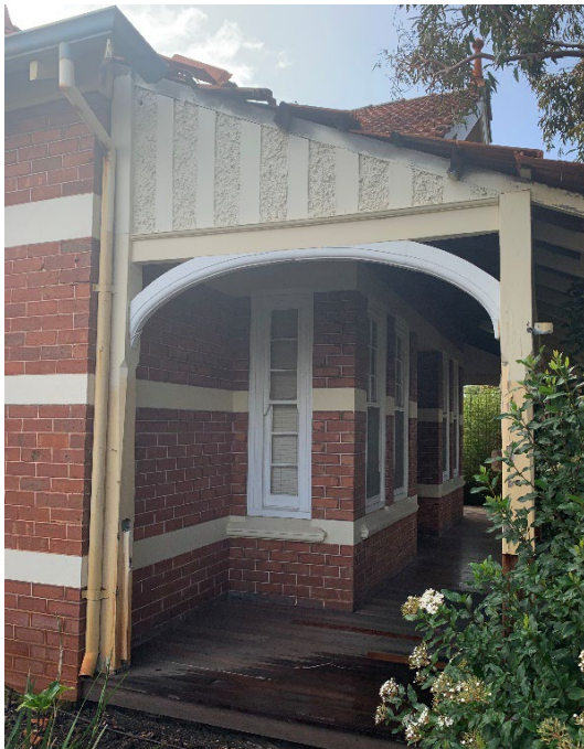
Figure 7: The brick walls to the front and side facades are tuckpointed and feature three rendered bands at sill, mid-window, and window head level, now painted (2024).
