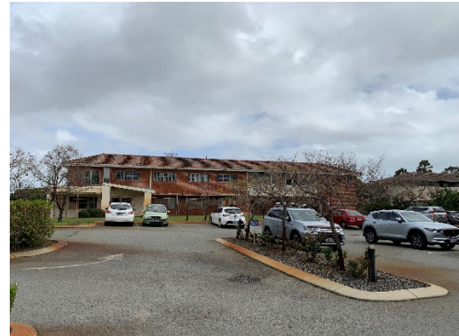
Figure 4: Wing located south-west of the 1920 Silver Chain building. These were constructed c.1956-57 (2024).
