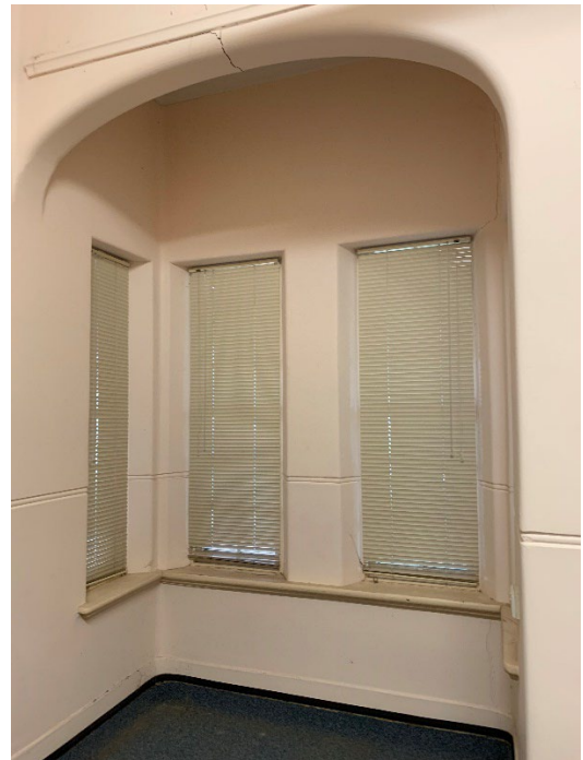
Figure 15: Internal detail of bay window, southern room (2024).
