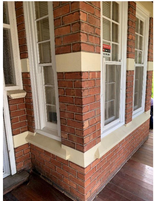
Figure 8: The bay windows consist of two double hung sliding sash windows facing the street, with smaller double hung sliding sash windows to each side of the bay window projection (2024).
