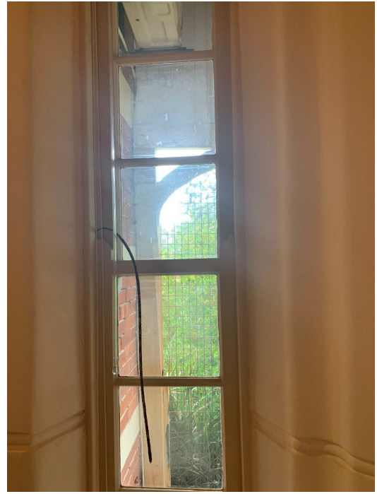
Figure 7: Double hung sliding sash windows on side projection of bay window. The frames and windows are likely original (2024).
