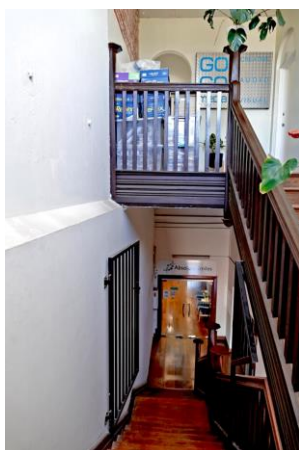
Figure 23. Front and rear entries to stairwell replaced c.1970s.
