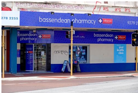
Figure 10. Shop front originally featured a central recessed entry flanked by large display windows. Replaced by current brick façade c.1970s, with a small display window and a wide raked entry at eastern end.
