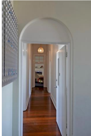
Figure 25. East-west corridor of Manager's Residence (2023) has polished timber floors, original timber skirtings and architraves (painted), rendered walls, and a 3.7m high flush ceiling with no cornices.
