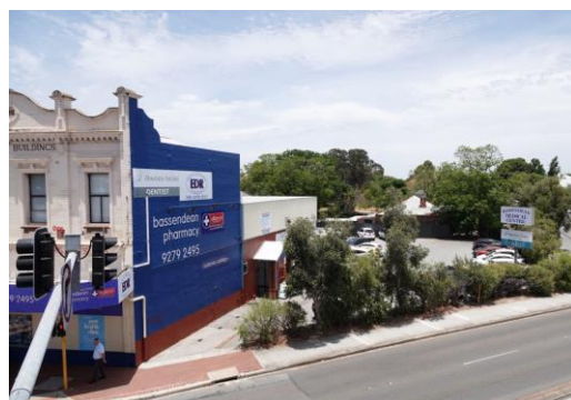
Figure 7. View of the carpark on the western side (2023).
