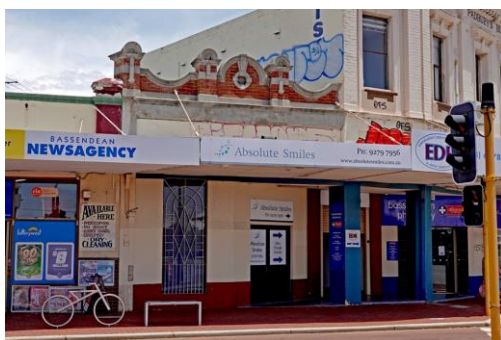
Figure 12. Form and detailing on ground level were extensively altered c.1970s. Original highlight windows above awning boarded up - unclear what remains under boards.
