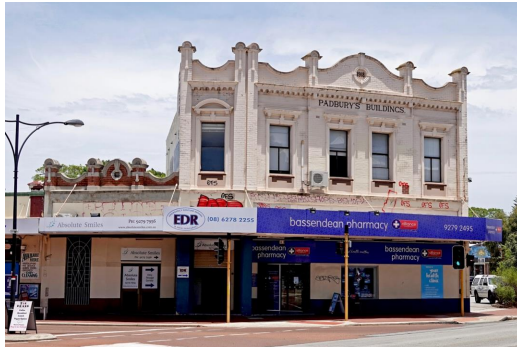
Figure 8. Visual impact of decorative detailing to first-floor façade diminished by painted finish. Original shopfronts significantly modified.
