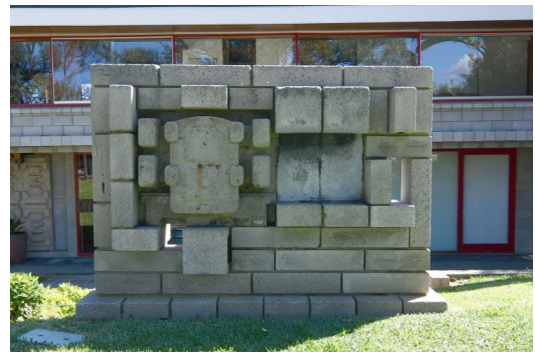
Figure 4: Original decorative concrete letterbox designed by Iwanoff for the house (front). Griffiths Architects 2023 .
