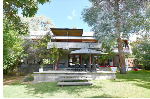
Figure 6: Balcony on the north facade. Griffiths Architects 2023.
