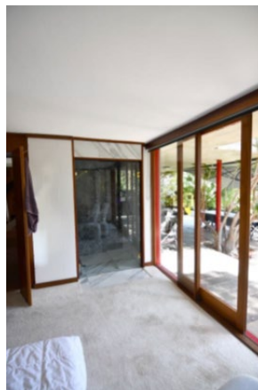
Figure 16: View of the master bedroom shower room connected directly to the bedroom. Griffiths Architects 2023.
