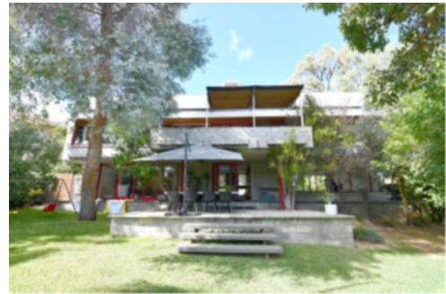
Figure 10: Balcony on the north facade. Griffiths Architects 2023.
