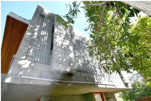
Figure 9: West elevation of the house. Griffiths Architects 2023.
