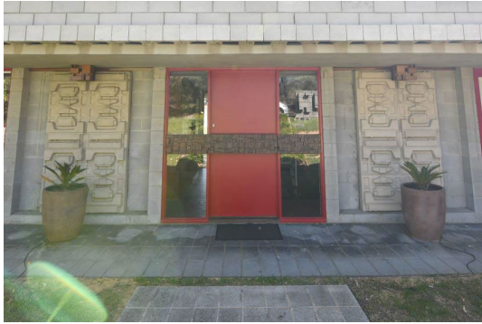
Figure 7: Front entry with decorative cast concrete panels and timber details. Griffiths Architects 2023.
