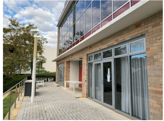
Figure 7: Front elevation ground floor. The doors are not original (June 2026).
