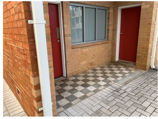
Figure 11: One of three ground level porches at the rear elevation (west). The central and west porch have the original terrazzo tiled floor. The location of the original brick partition wall (extant on the east porch, see Figure 10) is interpreted in the paving (June 2026).
