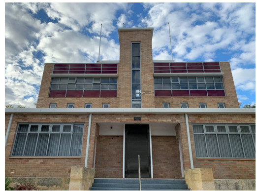
Figure 9: Rear elevation with curtain wall detail to the upper floors (June 2026).
