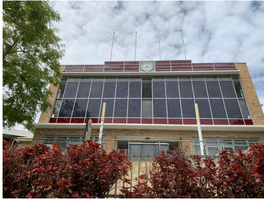
Figure 6: Front elevation from Stadium Drive. The flag poles are unlikely to be original as 1962 plans and photographs show three poles (January 2026).
