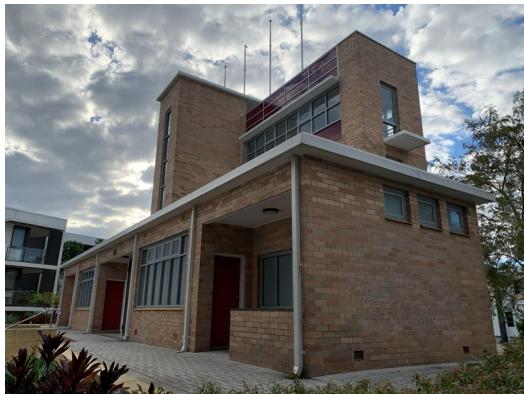
Figure 10: South east view of rear elevation (June 2026).
