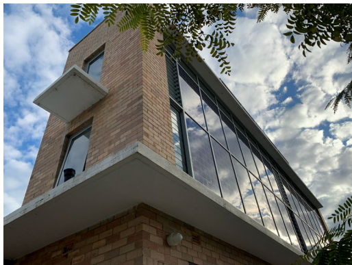
Figure 8: North east view of front elevation showing former viewing platforms (June 2026).
