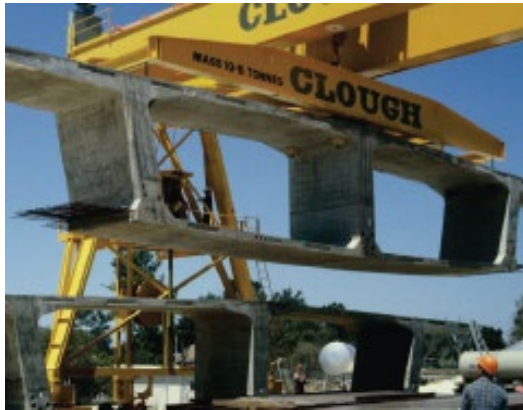
Figure 8: Original Mount Henry Bridge under construction. 43
