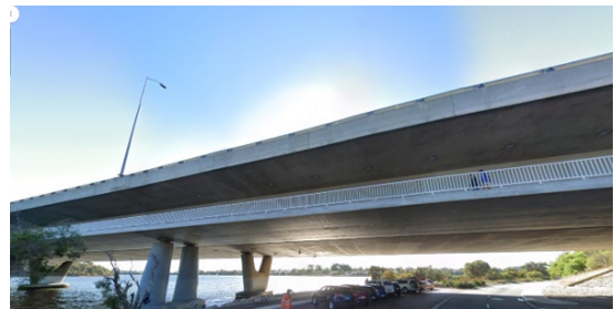
Figure 5: View from below bridge, west side, showing the 2007 bridge's double-column piers. 41
