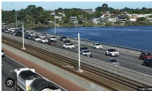
Figure 4: Mount Henry Bridge showing north and south bound lanes of traffic and rail lines in the centre. 40
