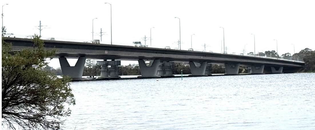
Figure 1: Mount Henry Bridge, viewed from the north, showing V-shaped original piers.
