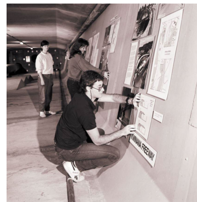
Figure 7: Inside the generous central utilities and maintenance void in Mount Henry Bridge . 42
