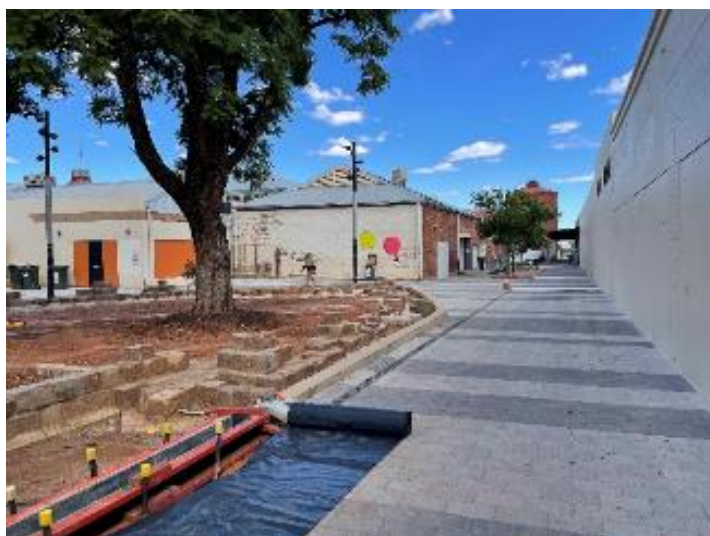
Figure 81. External View of St Barbara's Laneway
