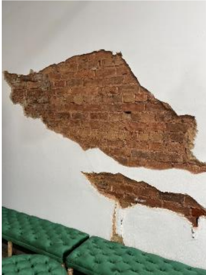
Figure 83. Detail view of No. 290 Damaged section of plaster render. It is unclear if this relates to historic rising damp or localised impact damage.
