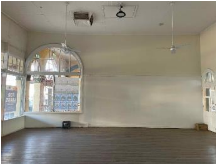
Figure 37. Internal View of No.272-280 Hannan Street, Tenancy 1
