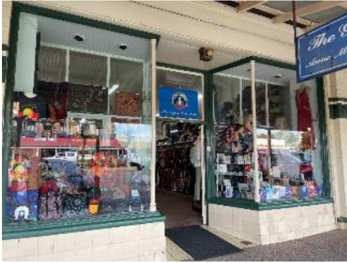
Figure 34. External View of No.270 Hannan Street
