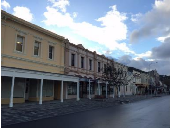
Figure 84. Stirling Terrace Heritage Precinct
