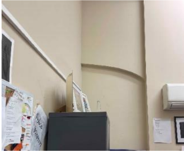
Figure 15. Internal View No.250-252 Hannan Street
