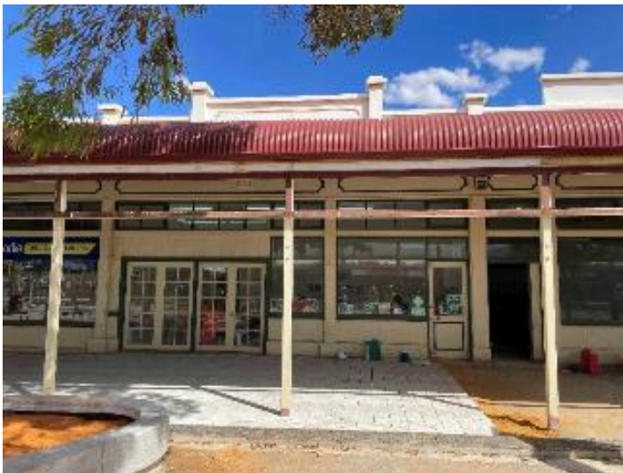
Figure 14. External View No. 250-252 Hannan Street.
