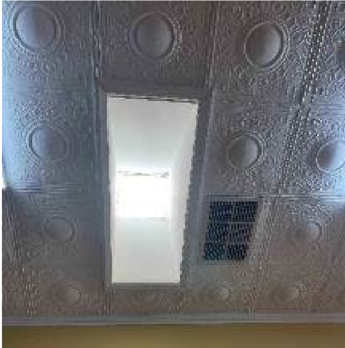
Figure 19. Internal View No. 256 Hannan Street.
