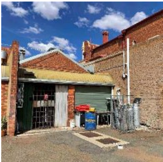
Figure 74. External View of No.312 Hannan Street The external verandah/courtyard opens out onto St Barbara's laneway, is fully enclosed, and used for storage.
