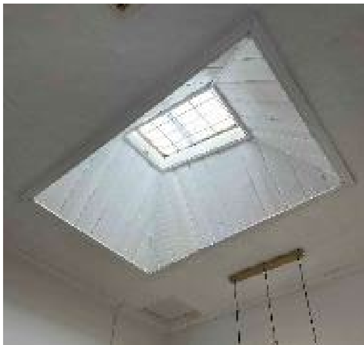
Figure 29. Internal View No.264 Hannan Street
