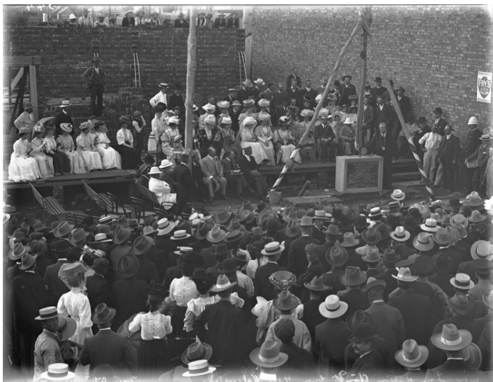
Figure 5. Laying the foundation stone of Kalgoorlie Town Hall, 6 November 1907. The foundation stone was laid by Mayor J.H. Cummins, in the presence of the Governor, Sir Frederick Bedford. State Library of WA, 010250PD
