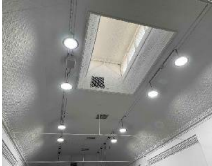
Figure 51. Internal View of No.290 Hannan Street
