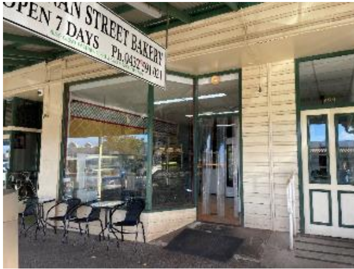
Figure 28. External View No.264 Hannan Street
