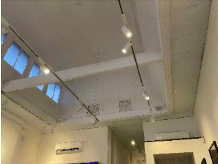
Figure 58. Internal View of No.296 Hannan Street
