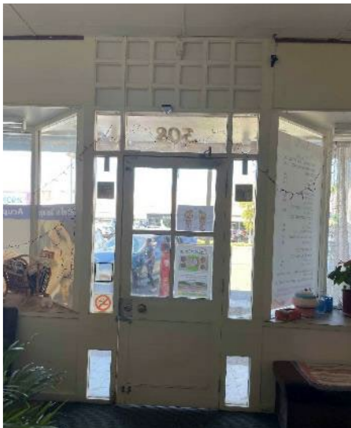
Figure 70. Internal View of No.308 Hannan Street
