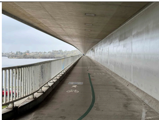
Figure 6: Mount Henry Bridge , from west side, showing shared pedestrian and cycle footway, cantilevered under the road bridge.
