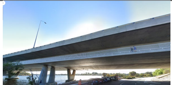
Figure 5: View from below bridge, west side, showing the 2007 bridge's double-column piers. 40
