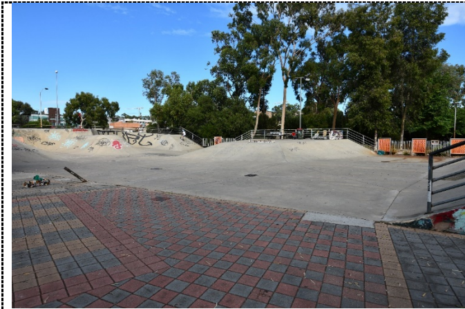
Figure 41. External view looking towards the Skate Park from the northeast corner.
