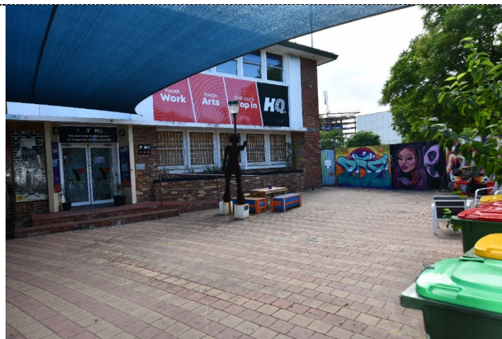
Figure 15. View of the courtyard showing main entrance. The timber double entrance doors have a fanlight above which has been covered over by signage. The original layout had a wind lock, but this has been removed. The ground floor brickwork of the central protrusion and base of western wall has tapestry brickwork the rest is in red brick.
