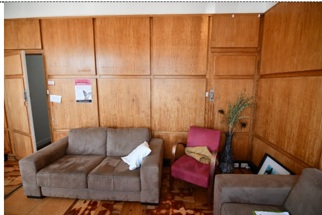
Figure 29. Interior Boardroom with original timber wall panelling original timber door panelling.
