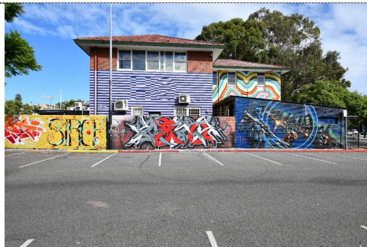
Figure 18. View of the east elevation of the Administration Building.
