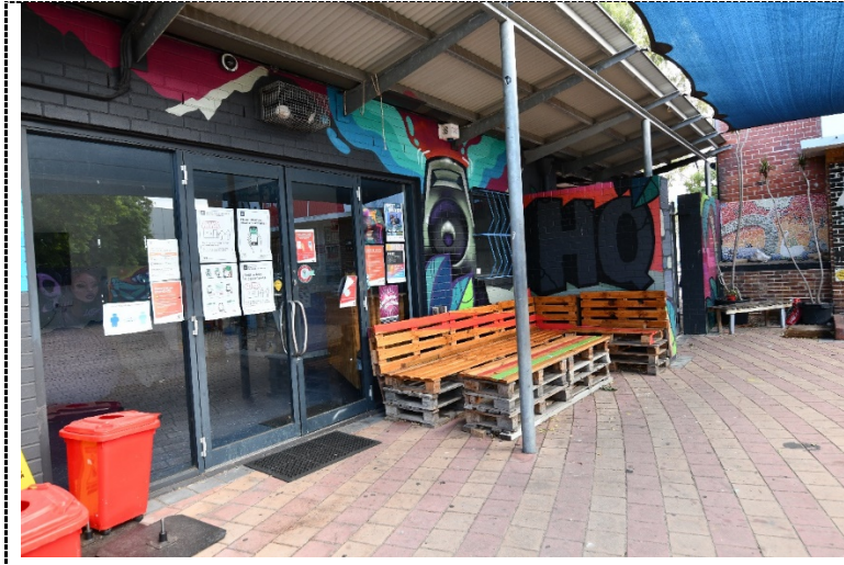
Figure 13. View of the HQ entrance from the courtyard.
