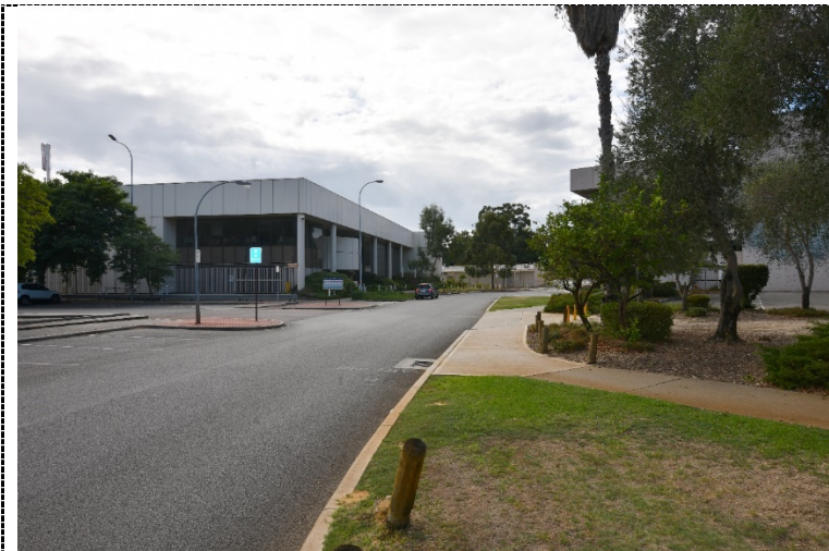
Figure 7. Commercial buildings and car parking sit to the east of the Administration Building.
