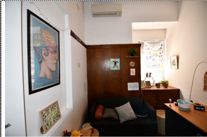
Figure 25. Interior Room 4 with original timber wall panelling originally a single room with Room 3.
