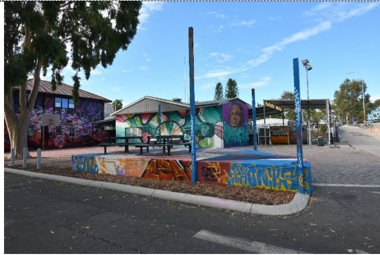
Figure 10. View of the Northern Elevation of the HQ Gig Space and Shed with Administration Building to the east.
