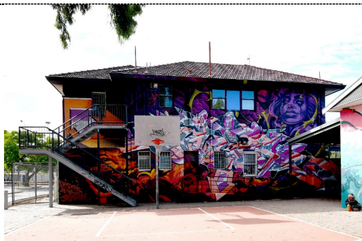
Figure 16. view of the west facade of the Administration Building with basketball court in front and HQ Gig Space to the south. The brickwork on the west elevation is covered entirely by graffiti artwork. An external metal staircase sits at the northern most end of the façade providing access to the first floor. A ramp provides access to the ground floor door. There is a mix of double hung sash and fixed windows on this elevation. The current external staircase is not original, and the orientation has been changed. Originally this staircase wrapped around the building terminated on the northern side instead of the west.
