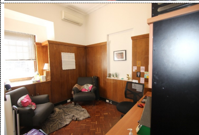
Figure 24. Interior Room 3 with original timber wall panelling and cupboard doors originally a single room with Room 4. The east window has been removed and blocked out, but the window remains readable.
