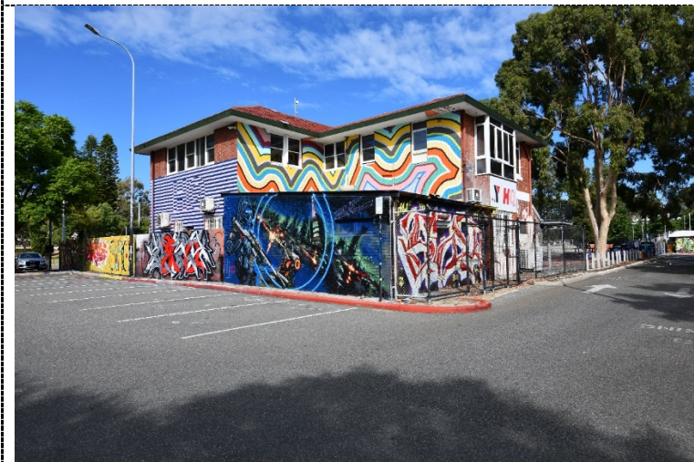
Figure 8. View of the northeast corner of the Administration Building and Toilet Block.
