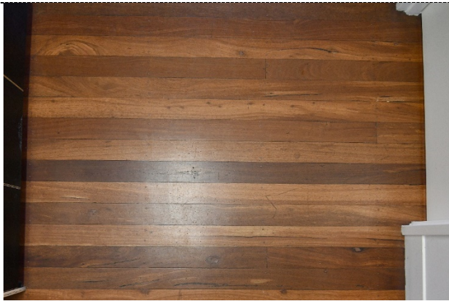
Figure 27. Interior view first floor hallway timber floor.
