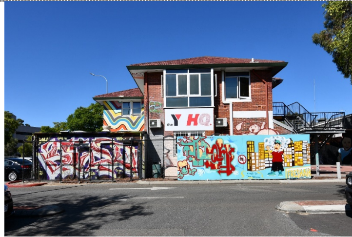
Figure 17. View of the north elevation of Administration Building and the later Toilet Block building and external staircase.
