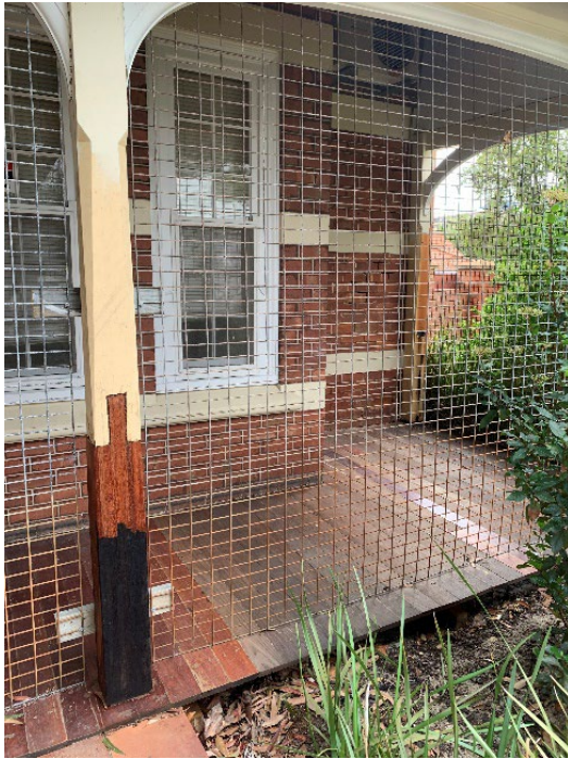
Figure 21: There have been sympathetic repairs to the timber posts at ground level. Security fencing has been installed inside the verandah to prevent unauthorised access (2024).
