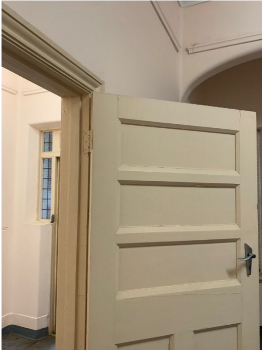
Figure 14: Detail of door and frame in southern room. The jarrah door frame is likely original, though the door is c.1950s (2024).
