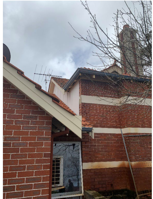
Figure 4: After the (c. 1920s-1950s) rear building was demolished in 1981, the gable roof was 'cut' and remnants of the connecting verandahs were retained. The rear verandah was then removed during construction of the current abutting building between 1995-2000. Board and batten panelling was installed to conceal the removal of the connecting buildings and verandahs.
