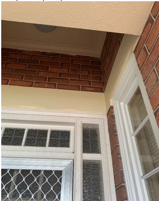
Figure 9: Detail to front door and right bay windows, with sliding sash window. The door is surrounded by hammered glass windows from mid door height and above (2024).
