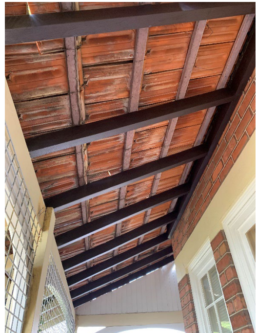
Figure 6: The roof is exposed rafter with simple curved timber frets (2024).
