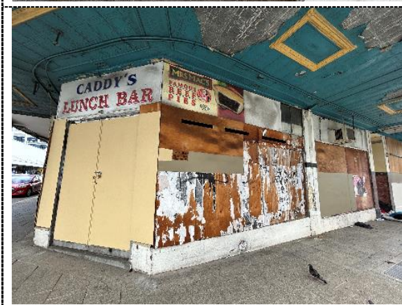
Figure 14. Large corner retail unit.
