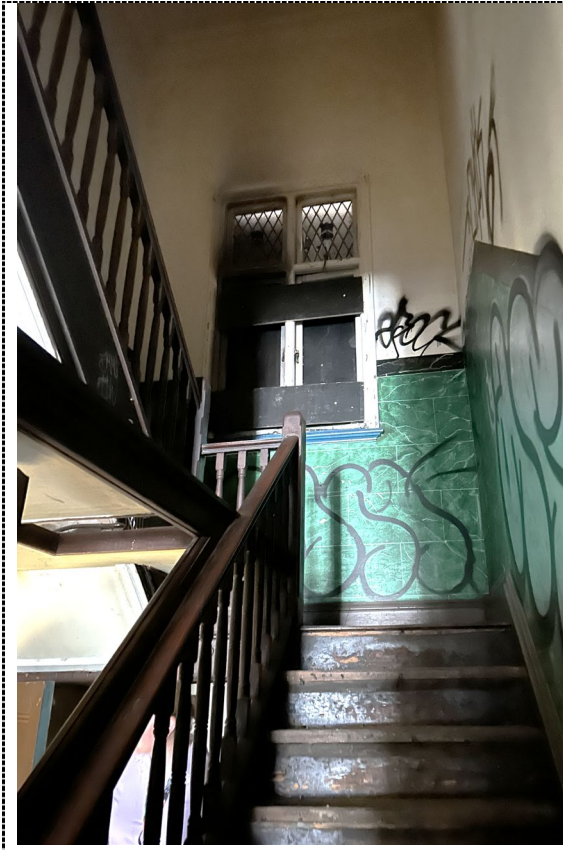
Figure 11 Original Pearl Villa staircase and mid-level landing.
