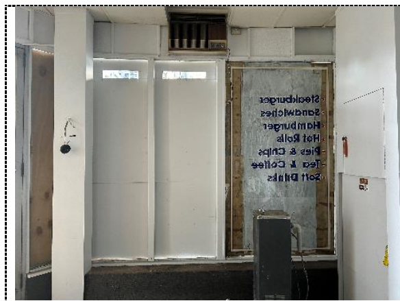
Figure 21. Non-original shop windows to the corner retail unit.
