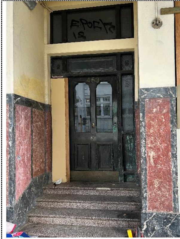
Figure 15. Main entrance into Milligan Hostel, Perth – original Pearl Villa entrance door which was relocated to the 1930s section.
