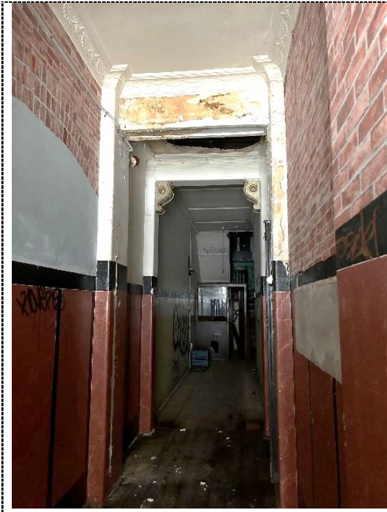
Figure 10 View from Murray Street entrance through hallway towards reception area.
