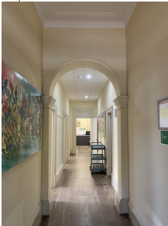
Figure 20: Front entrance hall with archway. The ceiling has been retained with original cornices and decorative ceiling plasters. False ceiling panels have been installed further along the same hallway and in several adjoining rooms. The hallway floor has been replaced, though original skirting boards have been retained (October 2025).
