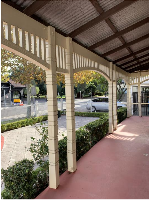
Figure 23: The verandah is painted concrete and has square decorative timber twin posts. Between the posts are arched timber valances. The verandah is unlined, with a single pitch roof (April 2025).
