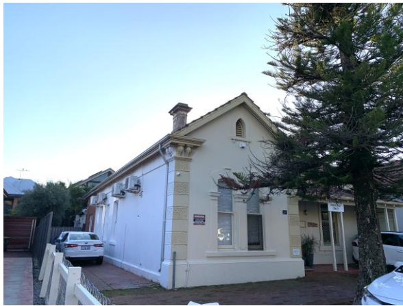
Figure 14: The façade of 122 Aberdeen Street features a single and twin set of double hung sash windows that are framed by heavy rendered moulding. A driveway runs to the rear of No. 122 (July 2025).
