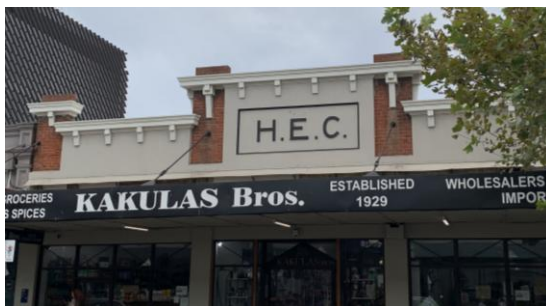
Figure 53: The building is face brick with brick piers to a stepped parapet that features the moulded lettering 'H.E.C'. 48 A flat awning, which has not changed form since all three previous tenancies were combined, features the store's name (February 2025).
