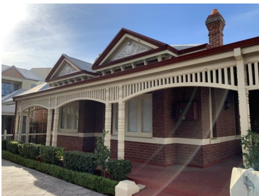
Figure 21: Stretcher bond faced brick with tuck pointing characterises the south elevation. There are two projecting bay windows with painted, rendered sills. The corrugated iron roof is a gable and hip roof, featuring twin gables with decorative painted render infill. Rendered brackets sit below the gables and eaves, and the eaves have timber slats to the underside. There are four brick and rendered chimneys with terracotta pots atop (April 2025).
