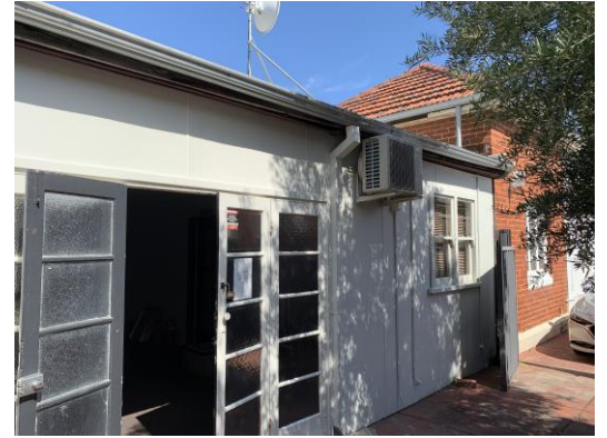
Figure 17: A rear extension was built over several phases, and the rendered brick portion is likely the original extent of the building (c.1897). Two brick extensions, one serving as the former kitchen (not pictured), were likely built around the same time (pre-1954, possibly 1930s, with modifications). The former kitchen was re-roofed in c.1974. The plasterboard enclosure was built c. 1981 and connects to the c.1930s brick kitchen extension and opens to a rear courtyard (October 2025).
