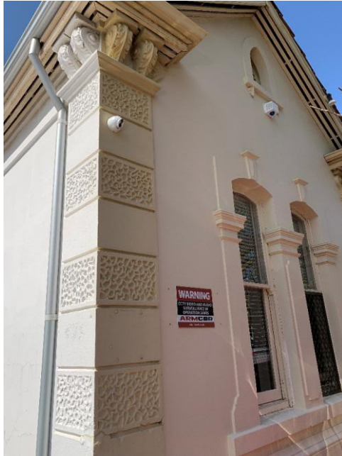
Figure 16: The façade of No. 122 features stone quoining with alternating bands of plain and vermiculated rustication, which is consistent with No. 120 (October 2025).
