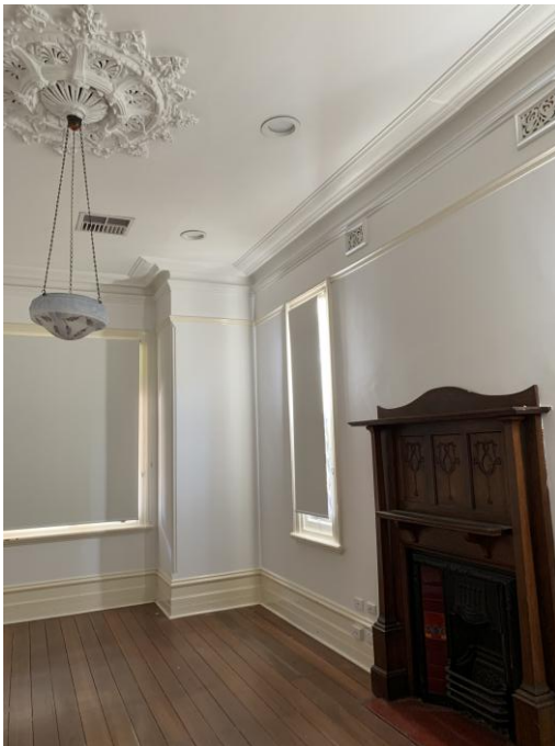
Figure 25: This room is the first door to the left of the entry hall. Notable features include timber floorboards, brick fireplace with timber surround, plaster ceiling with decorative cornices and ceiling rose, bay window and timber double hung windows, timber picture rail, and decorative wall vents (April 2025).
