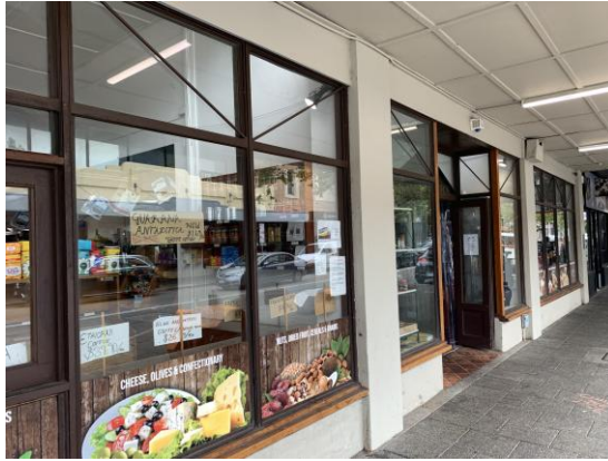
Figure 7: The shopfront is not original and was likely constructed when the tenancies were combined (c.1982-1993). Excluding the central entrance, each bay comprises three large, glazed window panels with three smaller windows above. Beams separate the bays which distinguish the original tenancies (February 2025).
