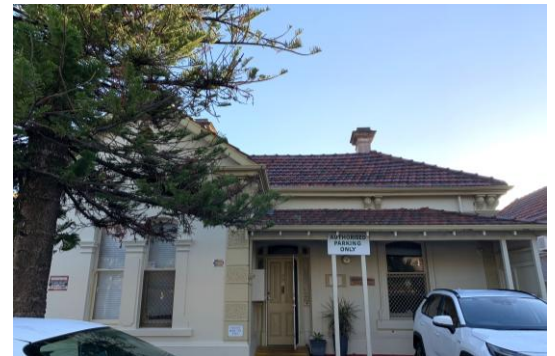
Figure 15: No. 122 has a porch verandah with a tiled roof and concrete floor. The eastern side of the verandah is enclosed with timber (c.1980s). Like No.120, the front door features side panels and leadlight windows (July 2025).
