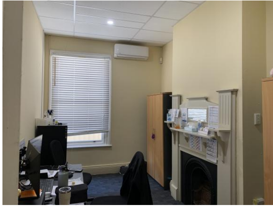
Figure 18: Example of room in c.1897 portion No. 122. The original fireplace and surrounds have been retained. Original floorboards are likely to be extant underneath the carpet. This room may have been part of an originally larger room, as indicated by the brick partition wall to the left of this image (October 2025).
