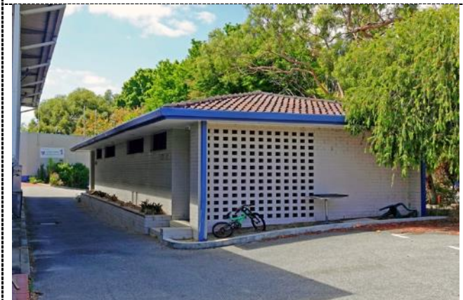
Figure 31. Toilet block (west) – north-west and north-east elevations
