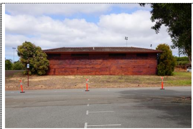
Figure 30. Toilet block (east) – east elevation
