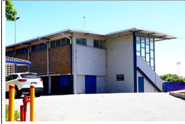
Figure 38. Velodrome grandstand – north-eastern elevation
