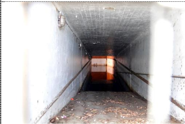
Figure 23. South-eastern end of cyclists' tunnel.
