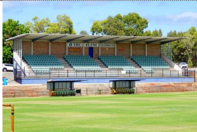
Figure 35. Velodrome grandstand – north-eastern elevation
