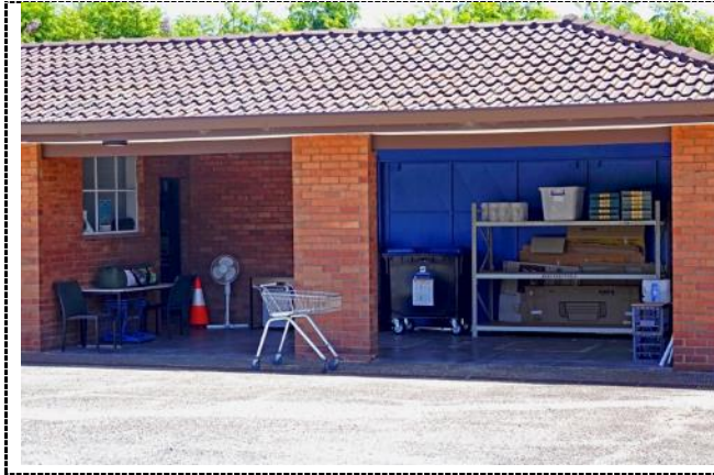
Figure 28. Turnstile/entrance building – eastern bay
