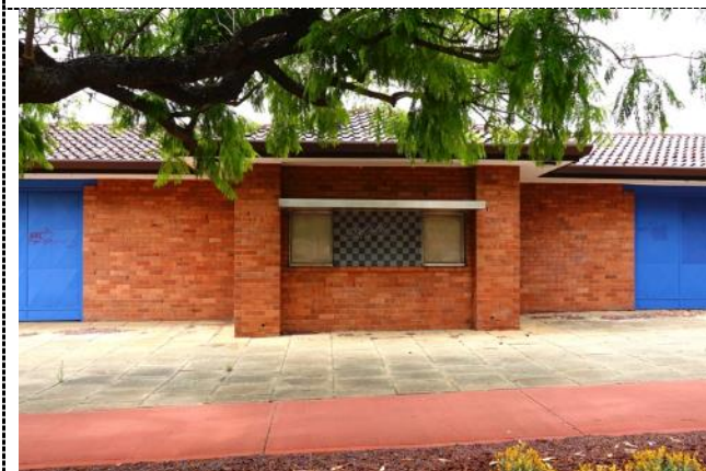
Figure 26. Turnstile/entrance building – north elevation – detail
