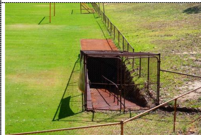
Figure 24. Reconfigured south-western entry to tunnel.
