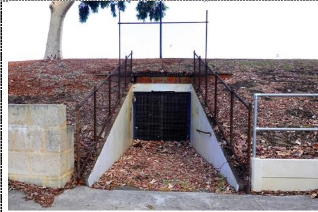
Figure 22. South-eastern entry to cyclists' tunnel.
