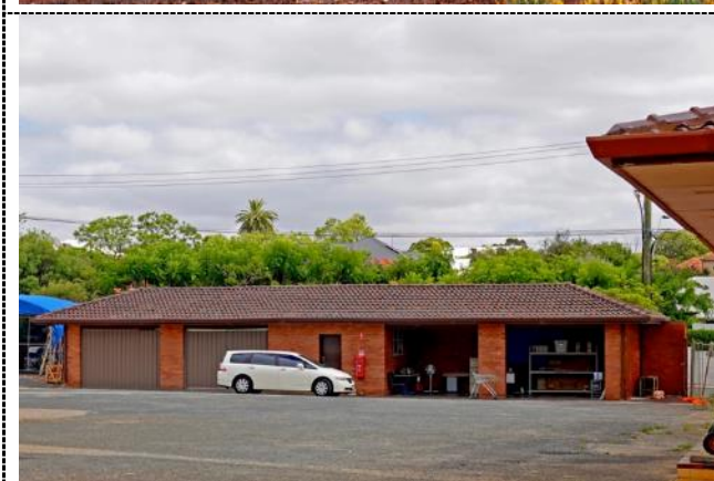
Figure 27. Turnstile/entrance building – south elevation
