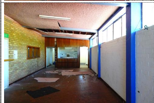
Figure 40. Function Room – reception area, looking south-east
