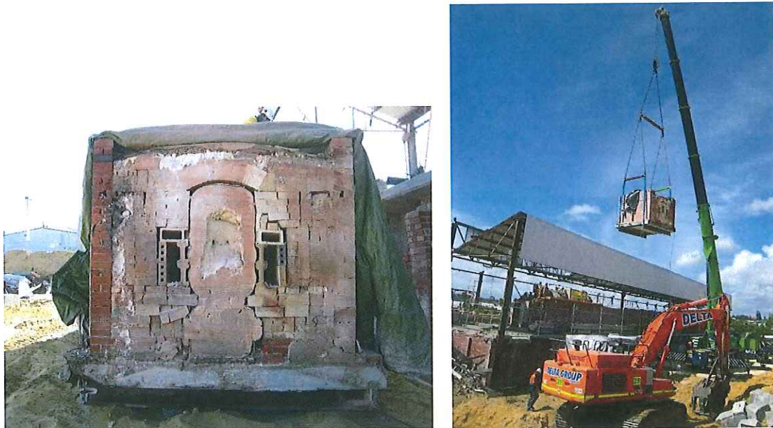
Figure 1.2 Section of tunnel kiln during relocation December 2010. The kiln void has been filled with expanding foam.
