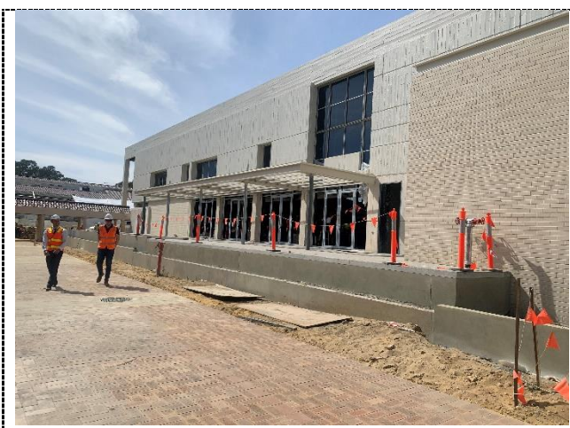
Figure 14. North Elevation Northern façade constructed in Béton Brut off-form concrete poured in-situ using pine to form a grain pattern. The upper portion of the façade is original fabric and remains extant. The lower colonnade has been infilled with new glazed entry doors and a glazed awning. The original columns remain extant. A furniture store, scene dock and new toilet entrance have been added.
