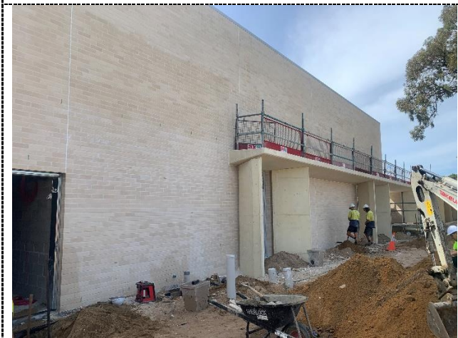
Figure 15. West Elevation Currently under construction, the new western addition is of tilt-up concrete construction with brick veneer, concrete fins and a concrete canopy. It will include male and female changerooms, drama and media studies staffroom, backstage area, external walkway, tech room, costume store and laundry, scene dock, furniture store and stage.
