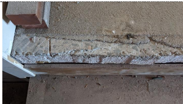
Figure 32. Original Flooring Detail in Bio Box Bridge
