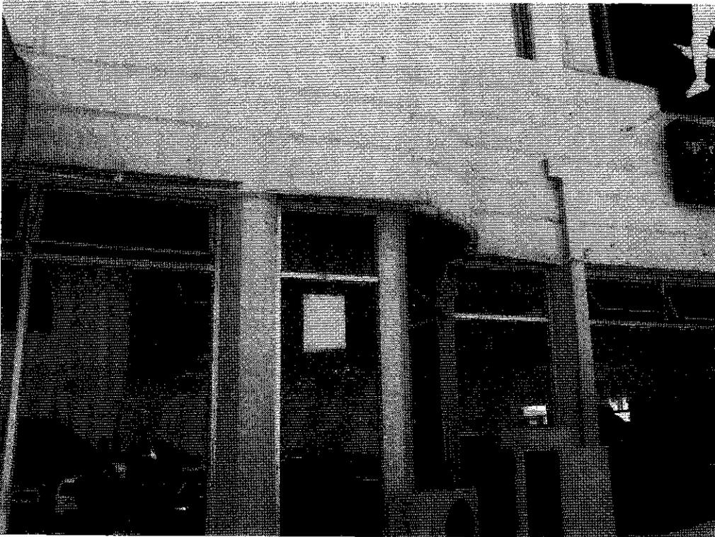
*Figure 108 Mirrored corner of previous image showing modifications to corner by installation of aluminium framed glazing. Hocking Planning & Architecture (WDW). February 2003.*
