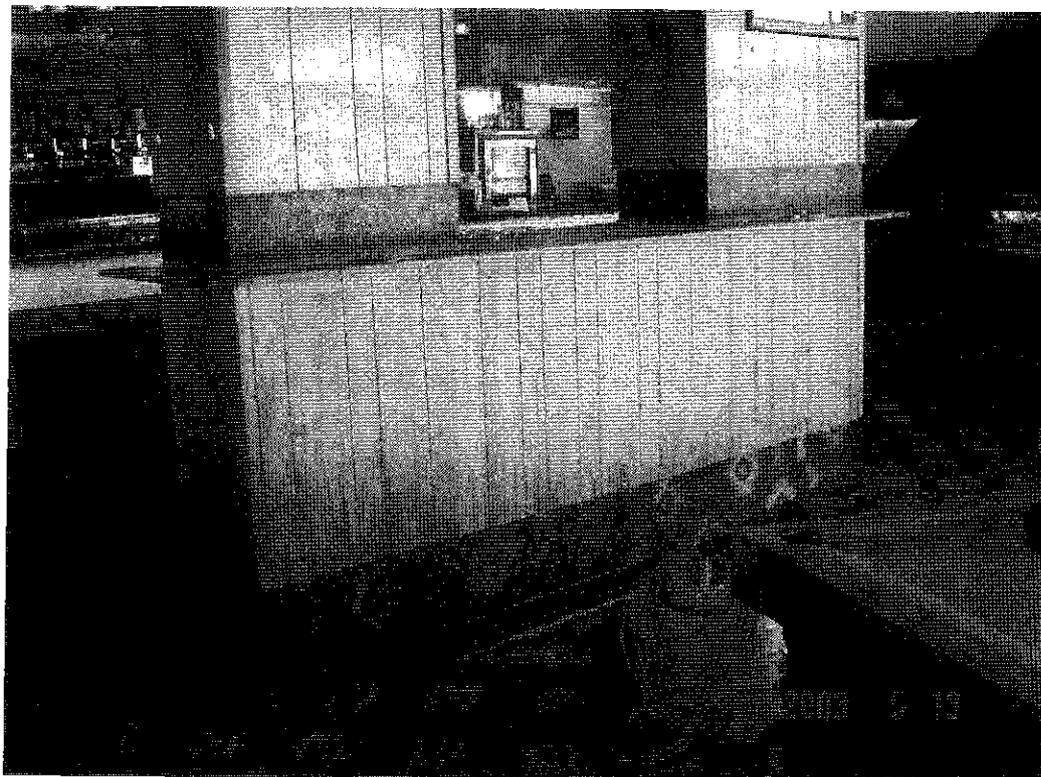
*Figure 113 Invasive investigation. Before – area of original 1896 external wall obscured underneath recent timber panelling. Mark Appleyard, Intonhouse Carpentry Services, May 2003.*
