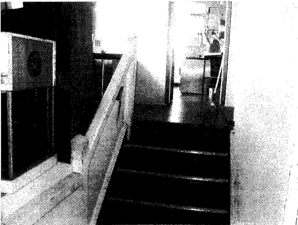
Figure 71 1937 timber and asbestos sheet service stair – note: only top flight is original. Hocking Planning & Architecture (WDW). February 2003.
