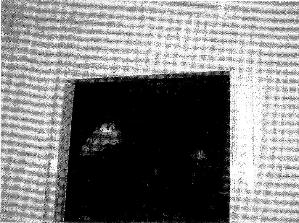
*Figure 56 Early door opening to dining room showing modified splayed architrave. Hocking Planning & Architecture (WDW). February 2003.*
