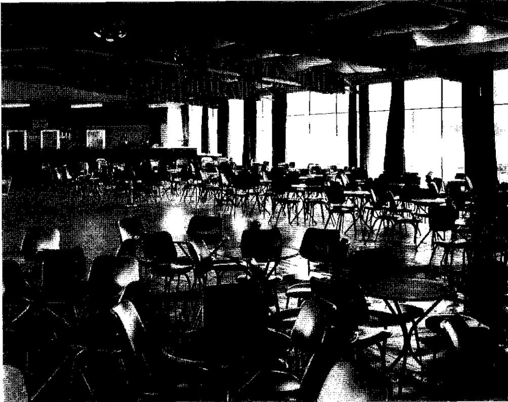
*Figure 26 The former open shed enclosed with glazed walling. The steel roof trusses are draped with fabric. Courtesy of Appin Investments.*
