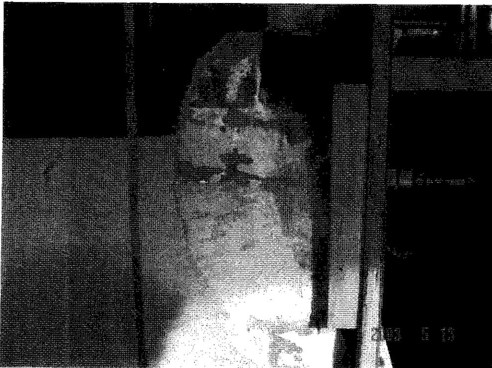
*Figure 117 Invasive investigation. After – section of 1896 wall paired down to show brick masonry with stucco banding overpainted with pale ochre. Mark Appleyard, Intonhouse Carpentry Services, May 2003.*
