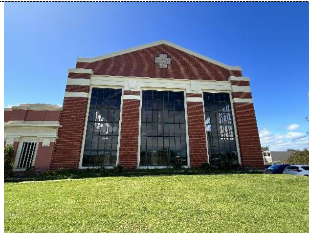
Figure 8. The large volume factory section has a classical presentation at the front elevation, with a classical balance of horizontal banding and vertical brick pilasters formed by the recessed vertical glazed panels under a gabled roof line.
