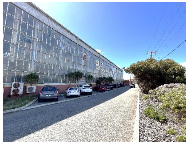
Figure 6. The southern side of the building is built hard to the boundary along Coventry Parade with angled parking along Coventry Parade.
