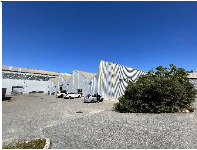
Figure 14. The saw tooth roof warehouse bays extend from the rear of the office section and were reduced in size in 2011. The distinctive roof form has been retained and the new east elevations have been clad with corrugated metal sheeting with two strips of translucent sheeting to each bay to allow for natural light. The southern plane of the roof form is glazed.
