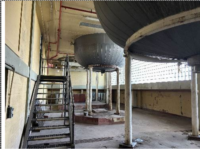
Figure 23. The underside of the brew chambers below the mezzanine floor.
