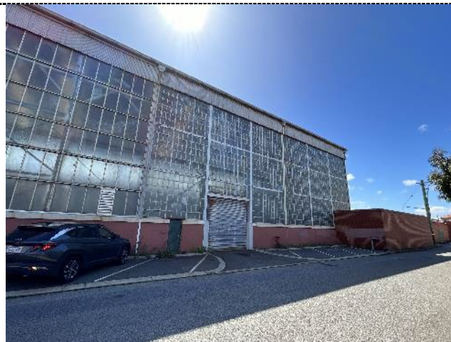
Figure 12. Contrast of glazing styles in the south elevation. The glazing panels to the 1930 section have been replaced with large rectangular panels with metal glazing bars.
