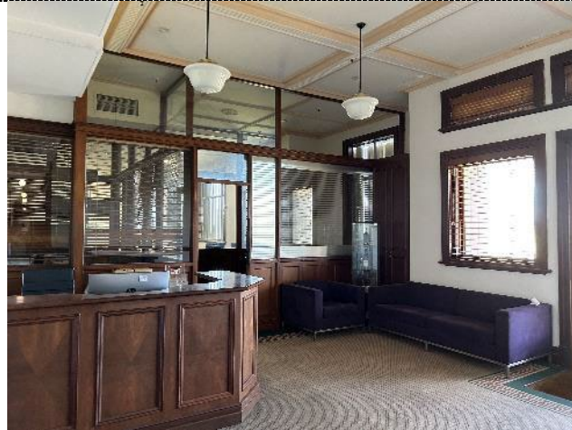
Figure 18. Reception/display area. The reception desk is not original although has been constructed to reflect the original timber partitioning of the offices. The ceiling is original.
