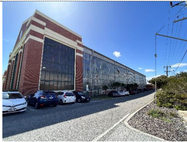
Figure 11. The south elevation of the large volume factory section is predominantly a glass curtain wall. The expansive elevation is effectively divided into bays by the prominent original rainwater heads. The fascia is corrugated metal sheeting.
