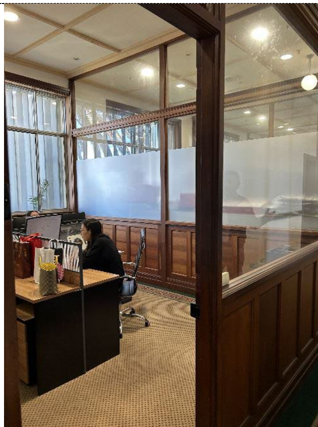
Figure 19. Typical office formed by timber and glazed partitioning. The partitions throughout the northern office area are a mix of extant and non-original. Changes to the details in the timber partitioning is evident in places, for example widths of timber panels and details on the architraves indicate that new material has been introduced and original fabric also altered to suit occupier requirements.
