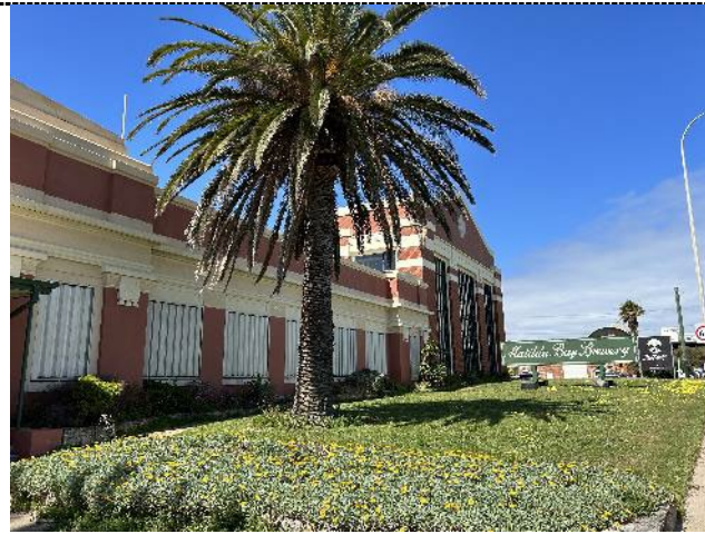
Figure 5. Palm trees and planting including green verge garden to the west of the building contributing to the green setting of the building along Stirling Highway.
